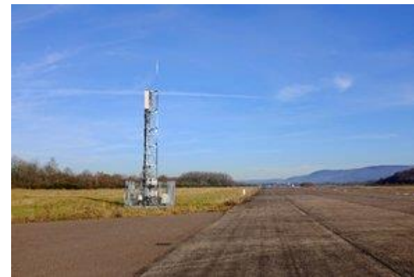
Towards 5G connected cars test runway
